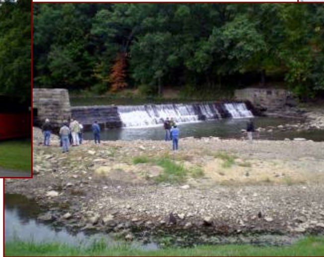
Bruceton Mill dam site
